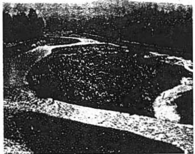
PHOTO 07-21. Set back levees on lower Tolt River allows the river to meander.
