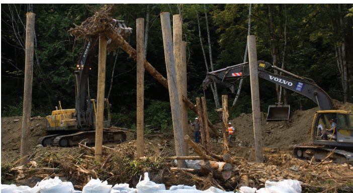
Logjam installation on Morse Creek
