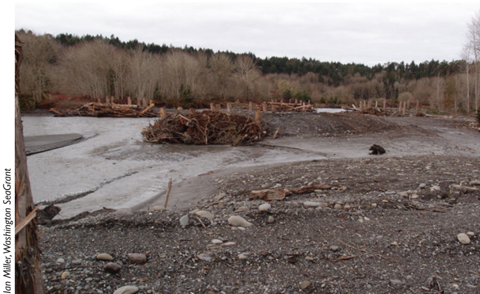
Newly constructed engineered logjams in the lower Elwha River. The structures are designed to split flows, activate new side channels, create pools and sort gravels.
