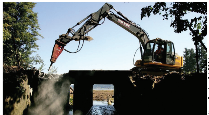
Workers pulverize Kittyhawk culvert.
