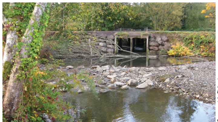
Kittyhawk Drive and culvert at mouth of Chico Creek, prior to removal of the road/culvert and restoration of the estuary.
