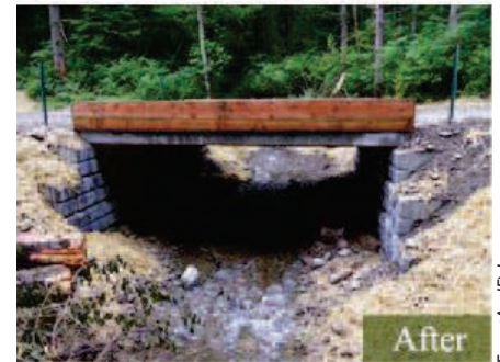
Example of RMAP road and culvert repair.
