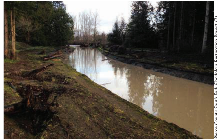
Completed South Fork Phase I Channel.
