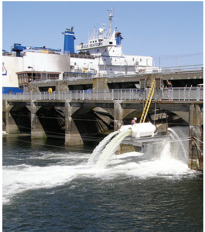
A ship moves through the U.S. Army Corps of Engineers' Ballard Locks as two smolt passage flumes (foreground) provide the only safe passage route to sea for juvenile salmon from the Lake Washington system. More fish passage improvements are needed, including replacement of 100-year-old lock valve machinery with new equipment to facilitate slower lockage fills that help reduce smolt mortality associated with navigation at the Locks.
